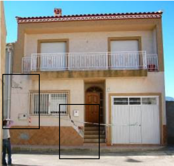
Moderate damage to infill walls in this home in Zarçilla. There appears to be slight damage to the column slab connection in the left hand photograph. (grade 3 vulnerability C)
