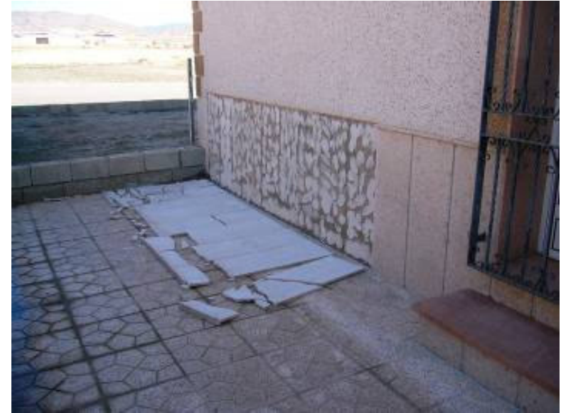
Different types of damage to decorative elements, balustrades and facing material in Zarcilla corresponding to damage of grade 2 across different vulnerability types.
