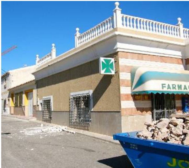
Different types of damage to decorative elements, balustrades and facing material in Zarcilla corresponding to damage of grade 2 across different vulnerability types.
