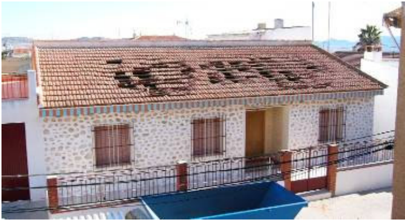
Damaged Roofs in various buildings in La Paca and Zarcilla
