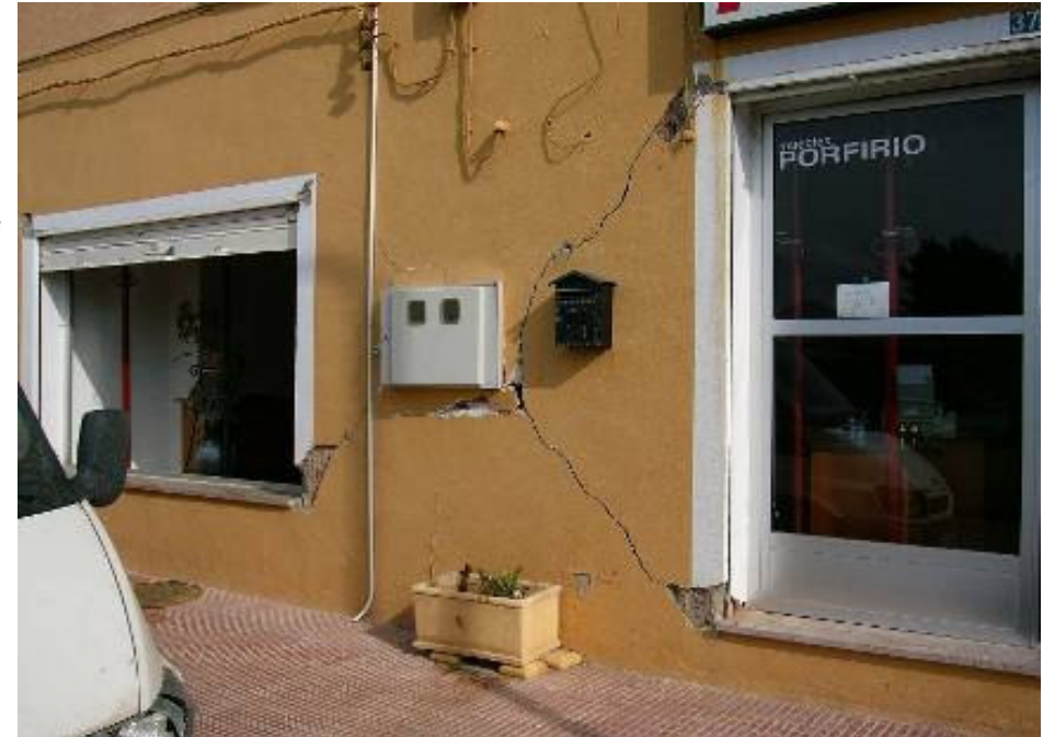
(left) shear damage in a building in Zarilla (Grade 2 vulnerability B)
