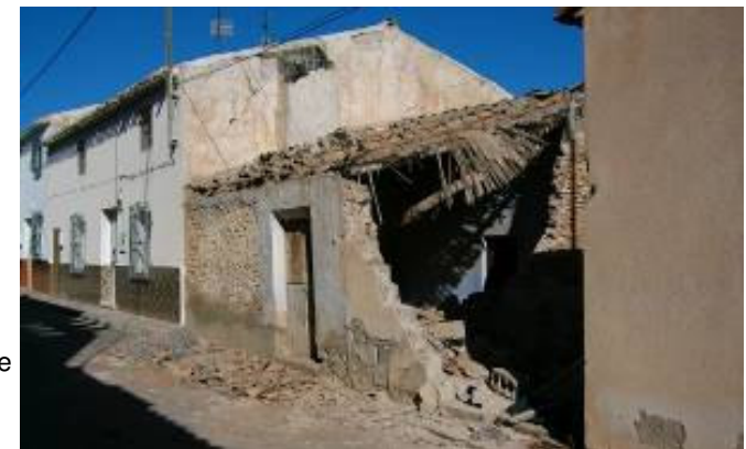
Corner failure. La Paca. (Grade 3 vulnerability A)
