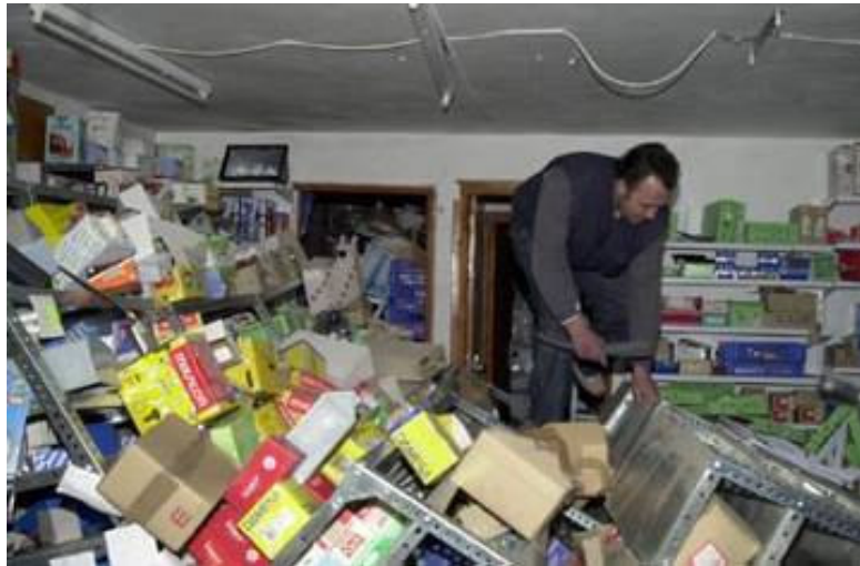
Toppled overloaded steel assembly racks in a hardware shop. Overturning of top heavy furniture is first used as a diagnosis for intensity 7. La Verdad de Murcia
