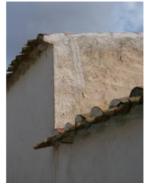
Very slight drift of load bearing masonry in masonry construction. Doña Inés (Grade 1 vulnerability A)
