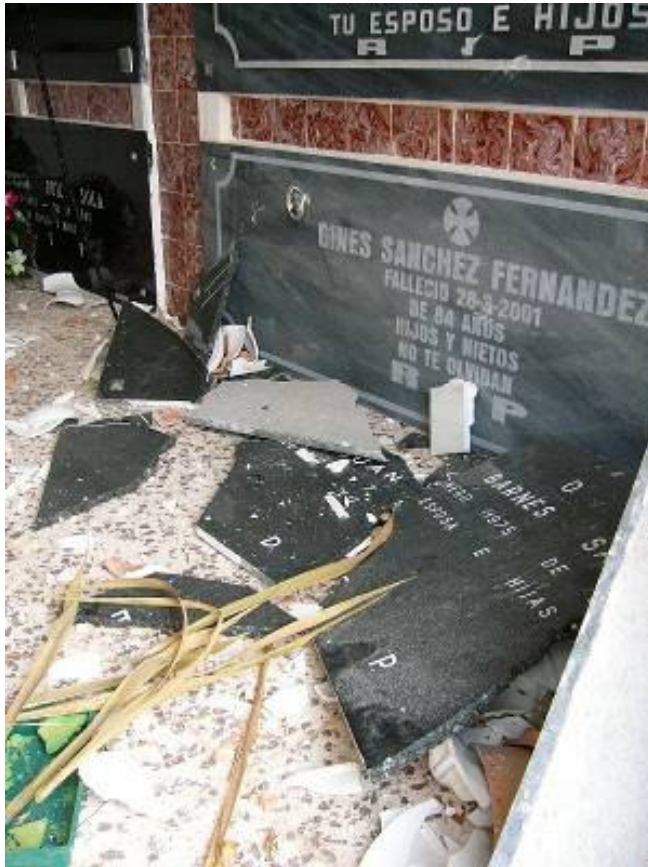
Damage to gravestones in Zarcilla
