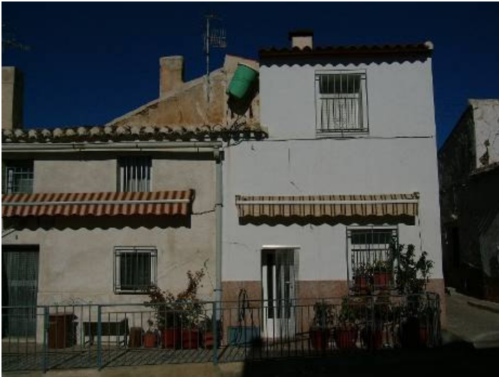
This water tank in La Peca was shifted, bending the plumbing connection and damaging the pedestal
