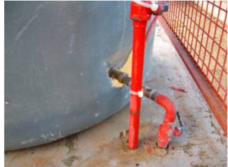
Bent and punctured connection, suggesting the tank was violently displaced in this direction.
