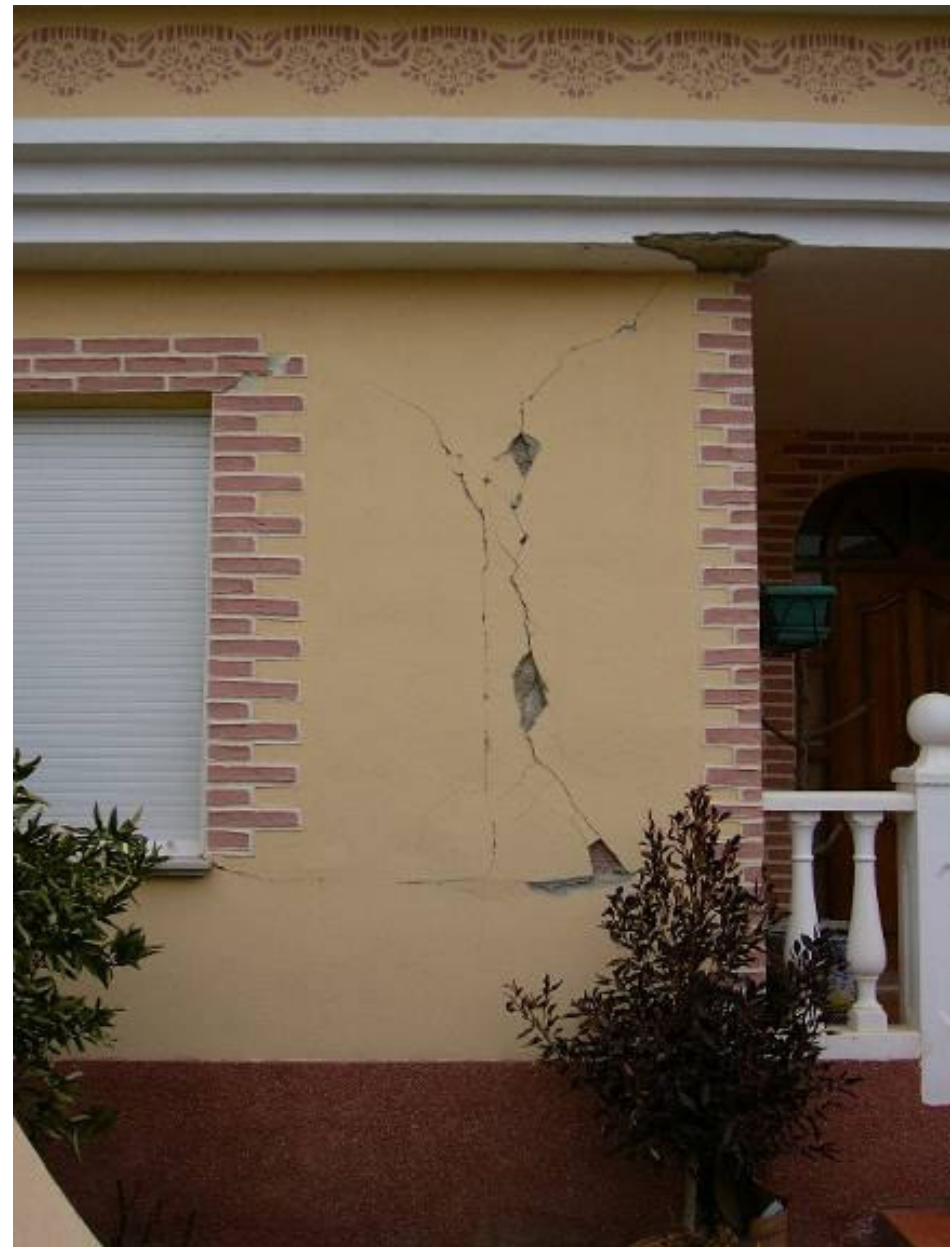
Moderate damage to infill walls in this recently completed home in La Paca (grade 2 vulnerability C)
