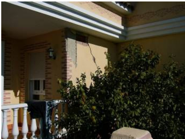
Moderate damage to infill walls in this recently completed home in La Paca (grade 2 vulnerability C)
