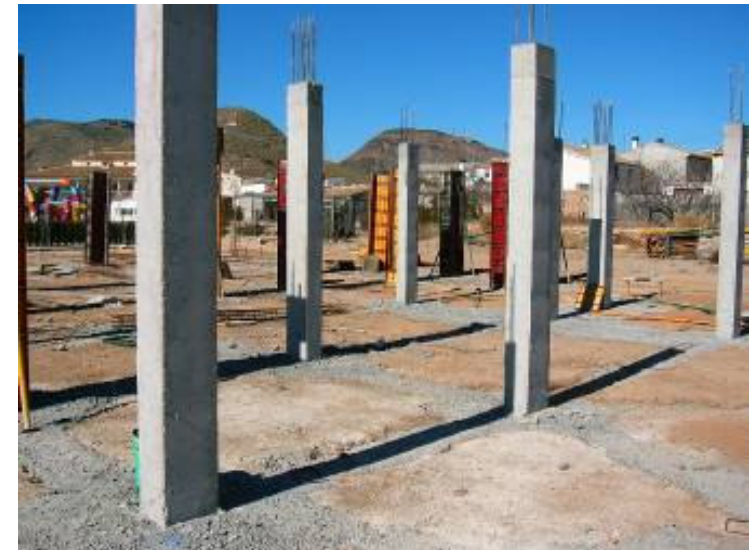
Modern construction systems for a housing project in Zarcilla, RC frames.
