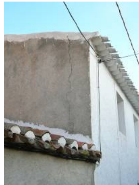
Very slight drift of load bearing masonry in masonry construction. Doña Inés (Grade 1 vulnerability A)
