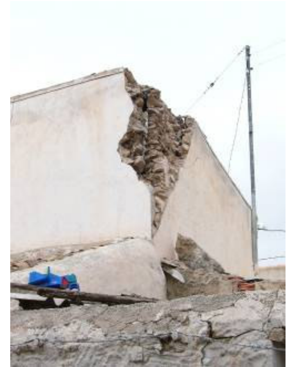
Corner failure. La Paca. (Grade 3 vulnerability A)
