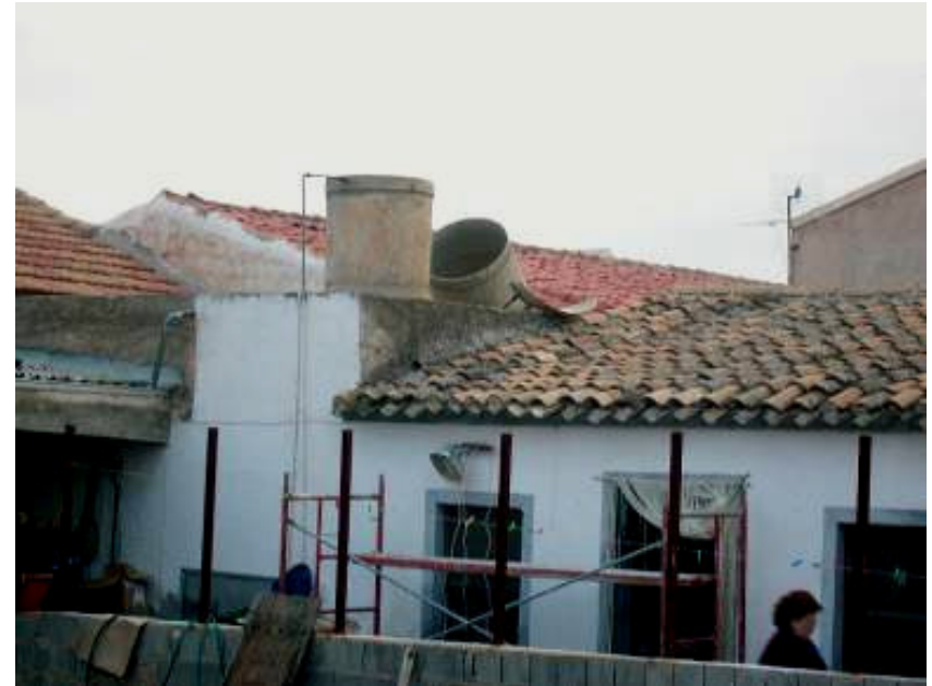
Overturning of a water tank in Zarçilla.
