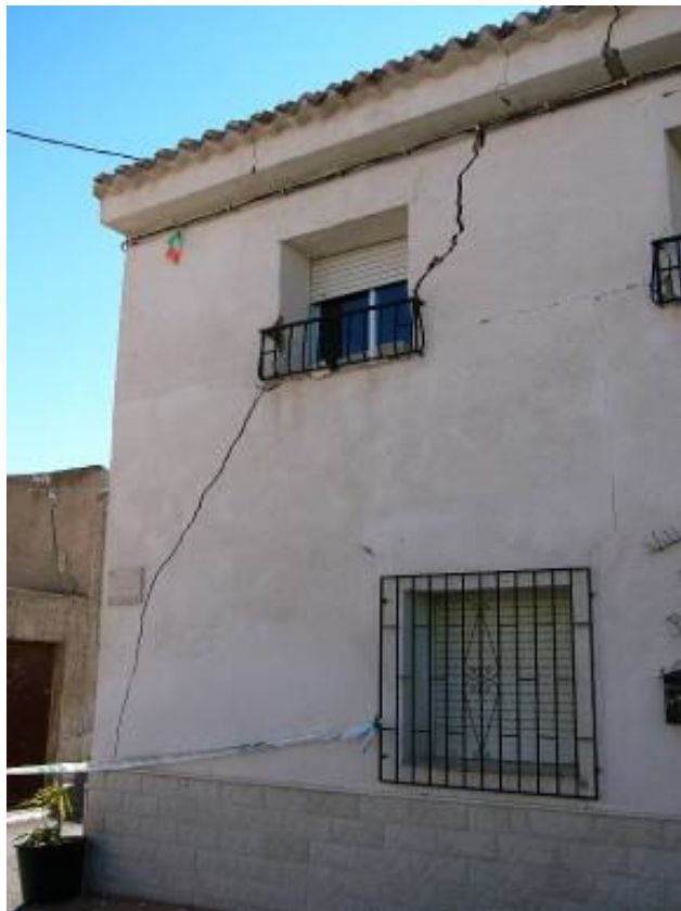
(left) shear damage in a building in Zarilla (Grade 2 vulnerability B)
