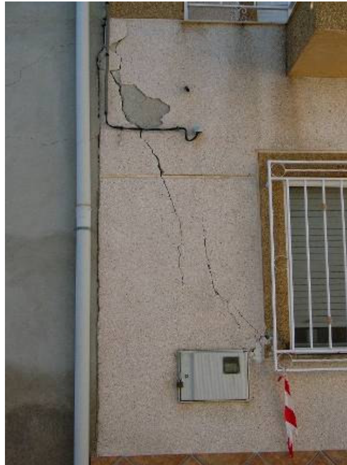
Moderate damage to infill walls in this home in Zarçilla. There appears to be slight damage to the column slab connection in the left hand photograph. (grade 3 vulnerability C)
