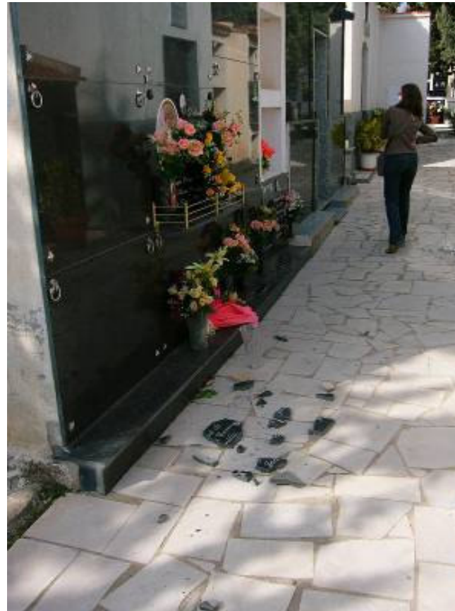
Damage to gravestones in Zarcilla
