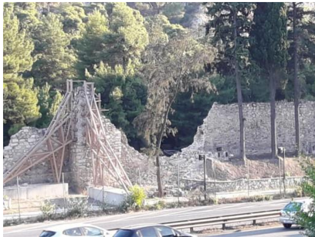
Figure 4. The position of the accelerograph (triangle) in the enclosure of the archaeological site of Dafni in relation to the site where the northern perimeter wall collapsed (star), the instrument installation and the wall collapse due to the earthquake.
