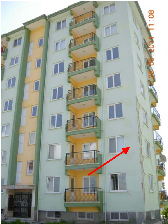
Figure 63: Damage at 7 storey rectangular building, spalling of concrete cover, widespread infill wall cracks
