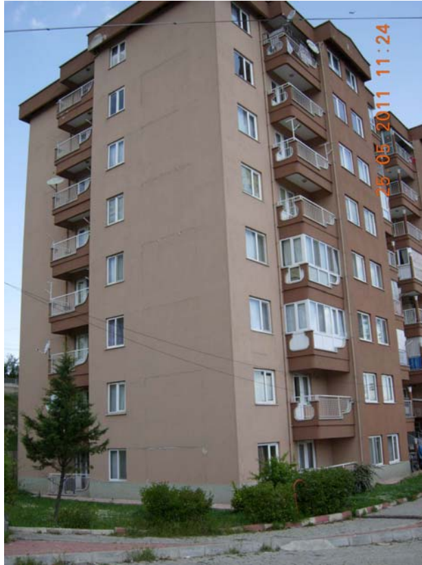
Figure 32: 8 storey rectangular buildings
