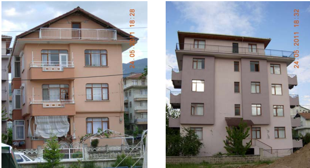
Figure 23: Simav town, typical 4-5 storey RC buildings -1
