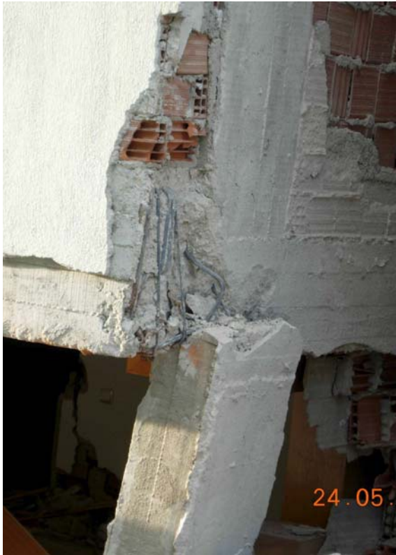
Figure 48: South-east corner column of the collapsed building
