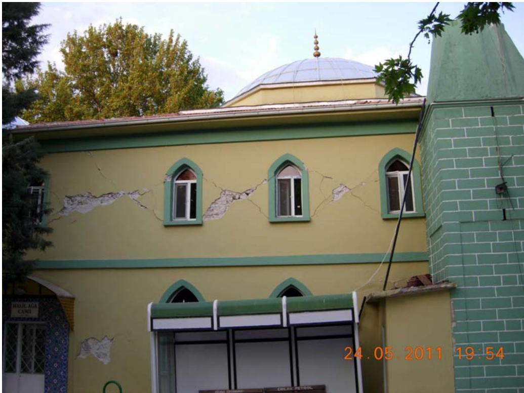
Figure 42: Brick masonry mosque, constructed in 1962
