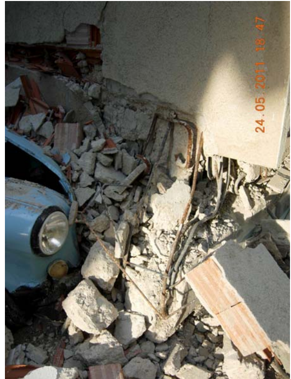
Figure 49: South-west corner column of the collapsed building
