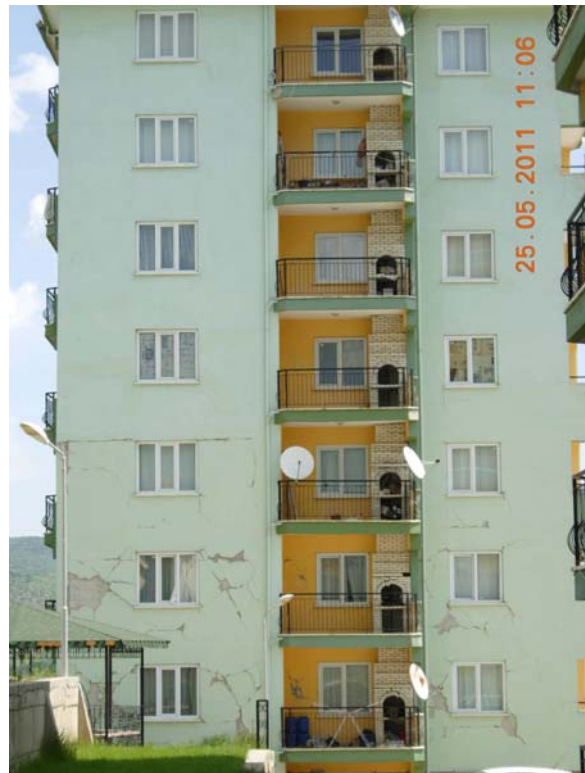
Figure 64: Damage at 7 storey rectangular building, moderate non-structural damage
