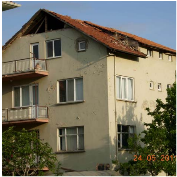
Figure 59: Roof damage
