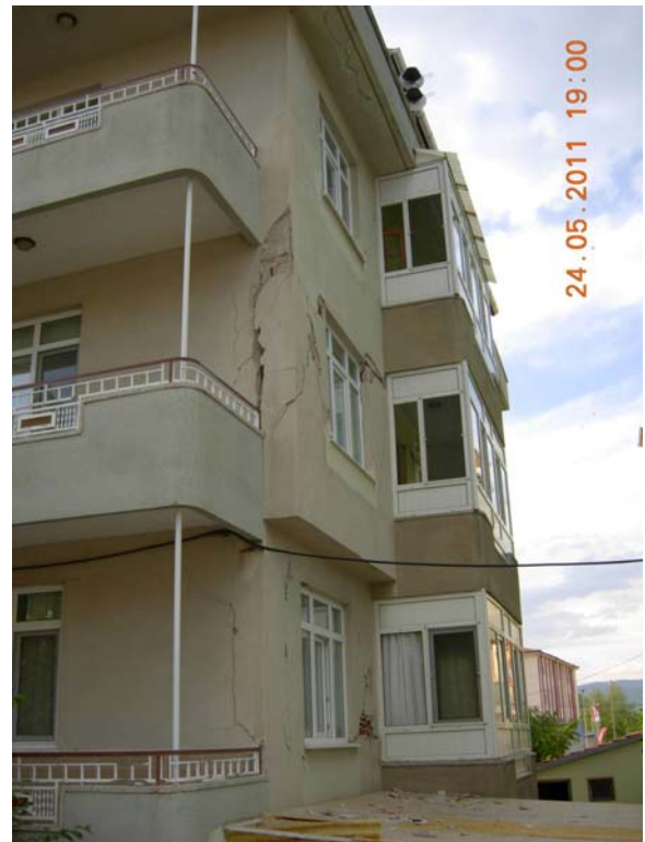
Figure 62: Damage at outer infill walls
