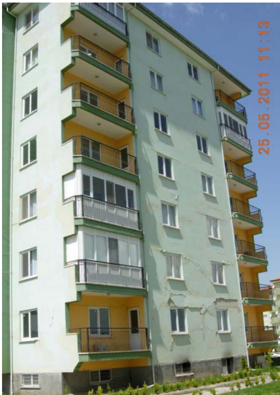
Figure 64: Damage at 7 storey rectangular building, moderate non-structural damage
