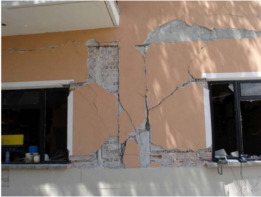
Figure 52: One of few examples for heavy structural damage, column behaved as a short column ,infill walls were composed of fired structural bricks instead of standart infill wall bricks.
