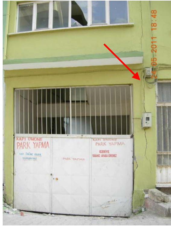
Figure 55: Damaged building, in front of the collapsed building, crack on the column extends from ground floor to roof.
