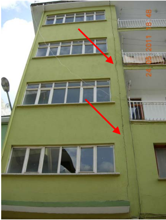
Figure 55: Damaged building, in front of the collapsed building, crack on the column extends from ground floor to roof.
