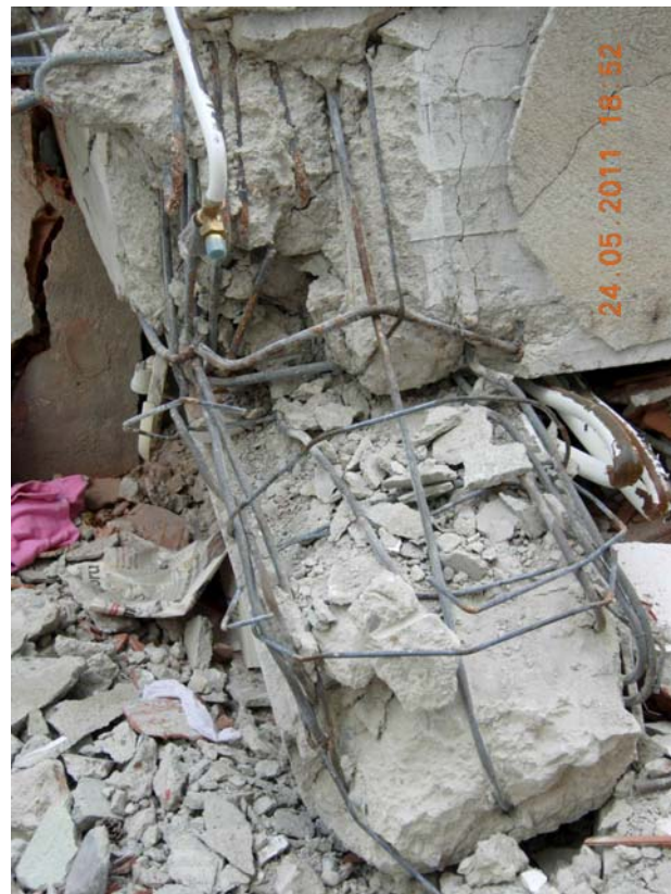
Figure 51: Beam-column joint detail of the north-west corner
