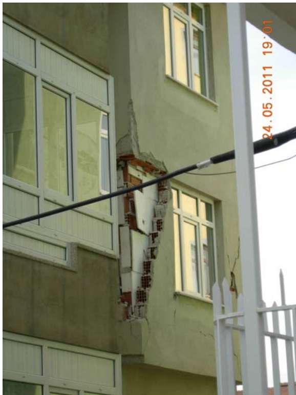
Figure 62: Damage at outer infill walls
