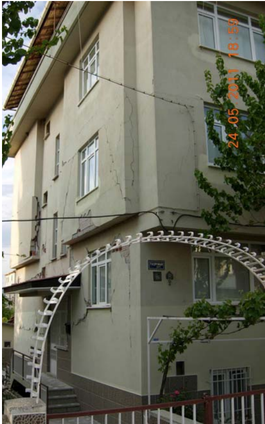
Figure 61: Infill wall damage and spalling of the plaster of structural members, front and side view
