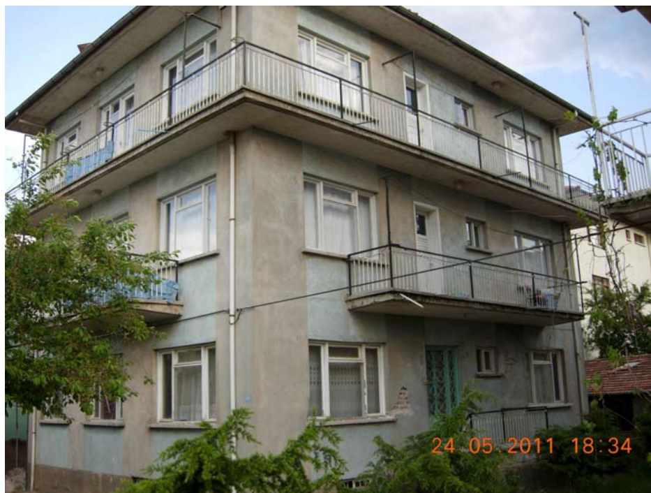
Figure 44: 3 storey brick masonry building
