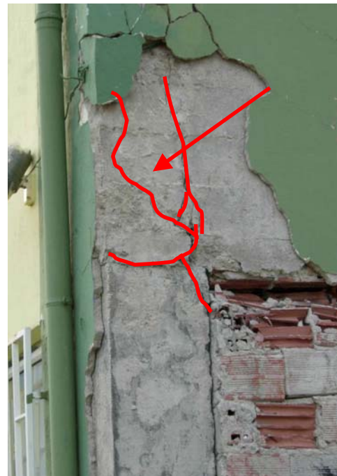
Figure 74: Cracks on beam-column joint of the RC part of school building
