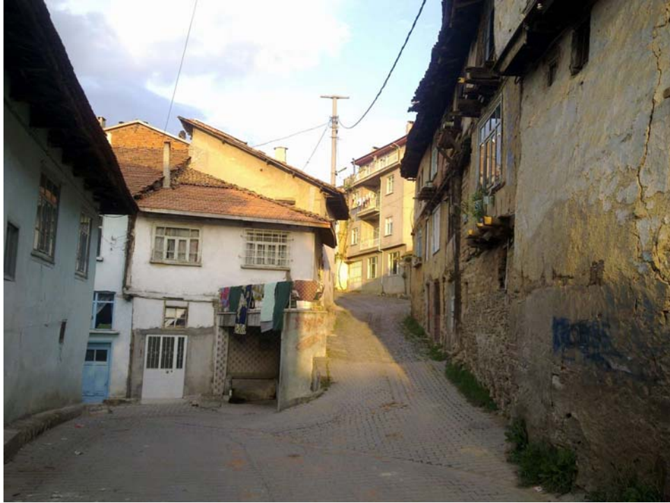
Figure 37: A street view, having adobe and brick masonry buildings - 2
