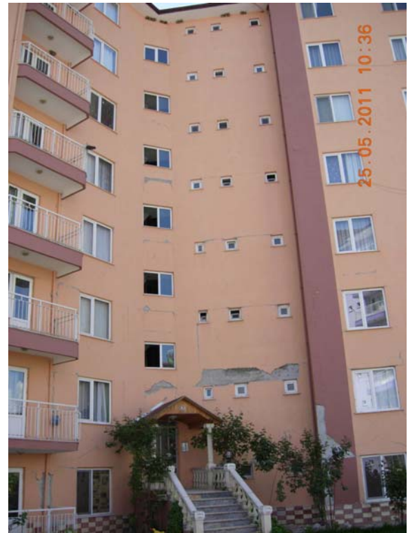
Figure 65: Damage at 8 storey star buildings, moderate non-structural damage
