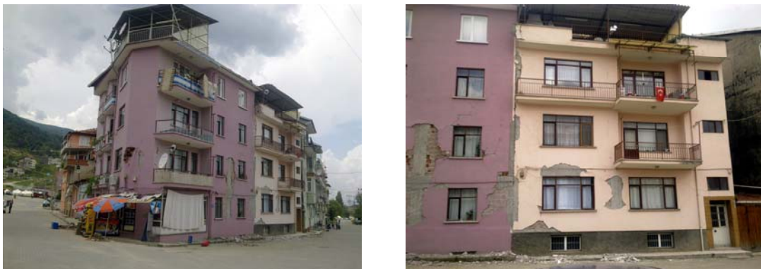
Figure 24: Simav town, typical 4-5 storey RC buildings - 2
