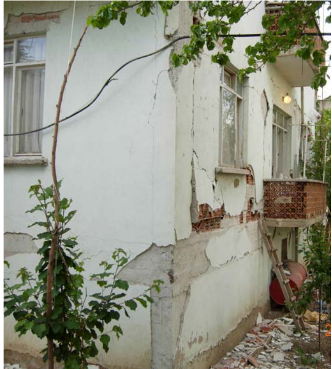
Figure 61: Infill wall damage and spalling of the plaster of structural members, front and side view
