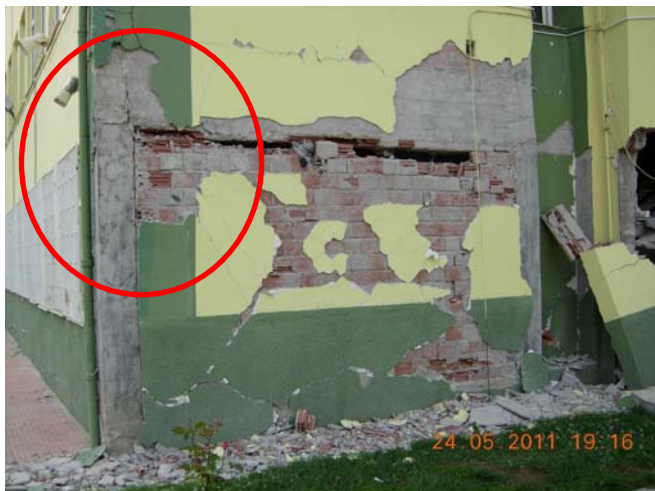
Figure 74: Cracks on beam-column joint of the RC part of school building
