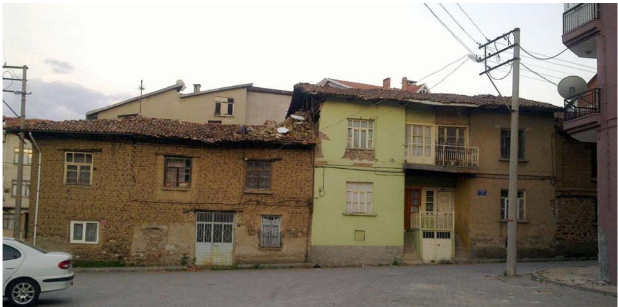
Figure 40: 2 storey adobe masonry buildings - 2
