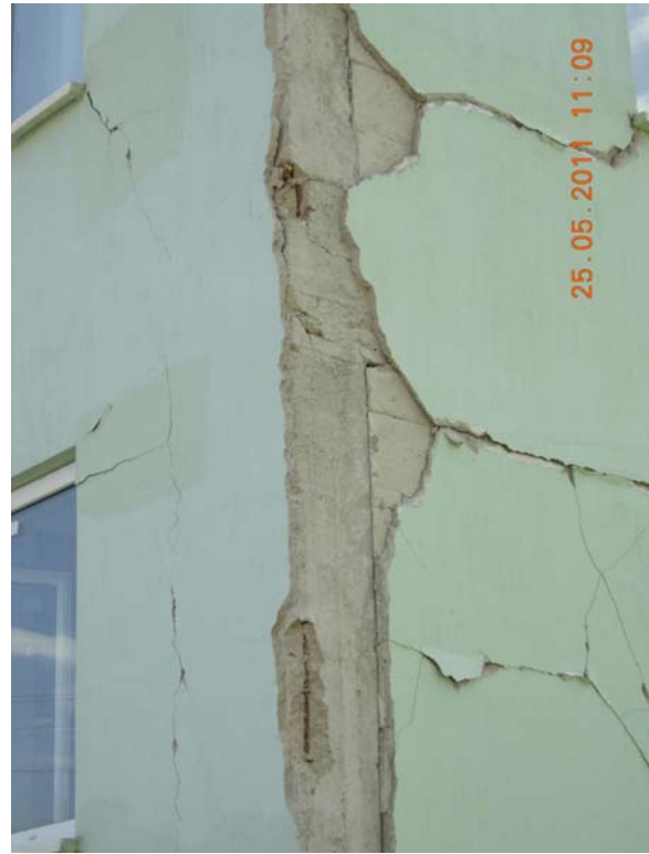
Figure 63: Damage at 7 storey rectangular building, spalling of concrete cover, widespread infill wall cracks
