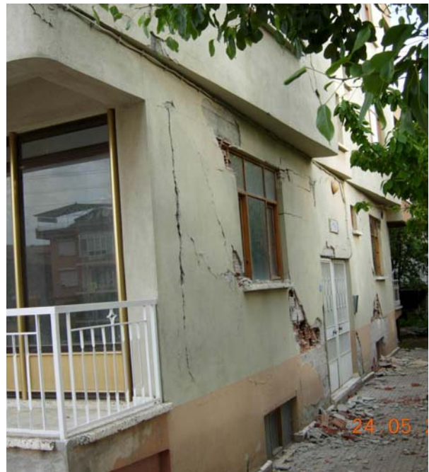
Figure 60: Infill wall damage, front and side view
